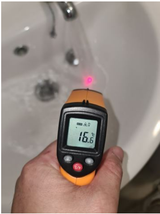
Image 2: Cold Water System
