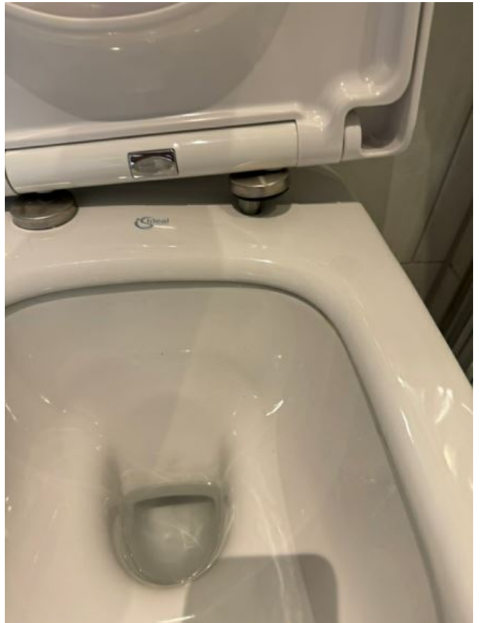
Image 68: ENSUITE SHOWER ROOM
