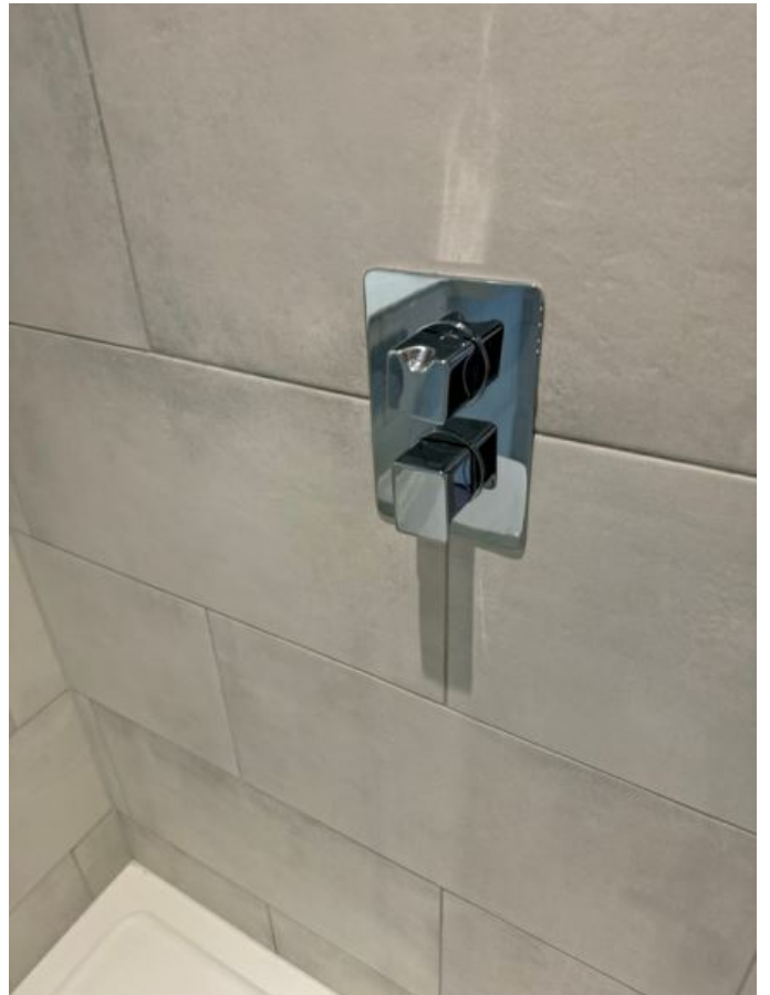
Image 60: ENSUITE SHOWER ROOM
