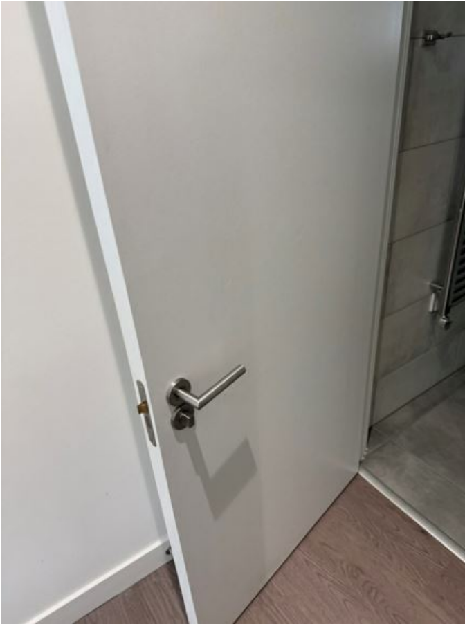
Image 55: ENSUITE SHOWER ROOM
