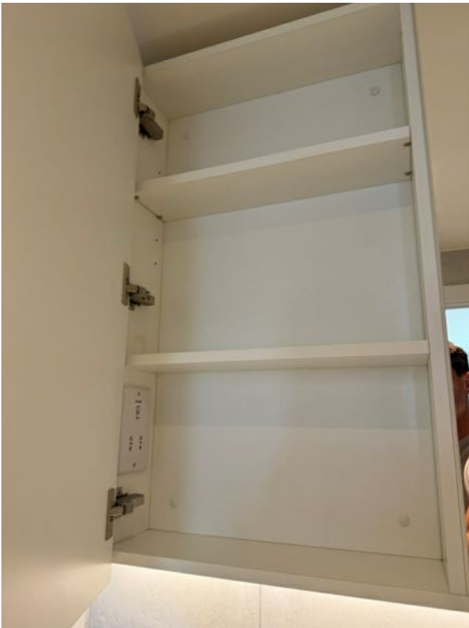
Image 71: ENSUITE SHOWER ROOM
