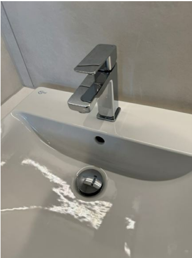
Image 69: ENSUITE SHOWER ROOM
