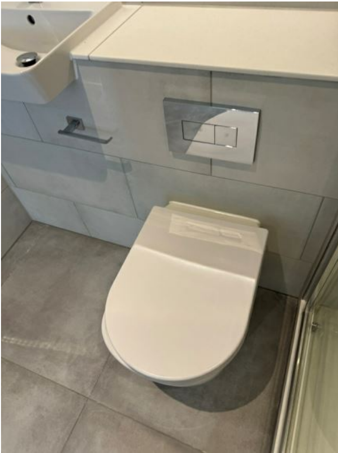
Image 63: ENSUITE SHOWER ROOM
