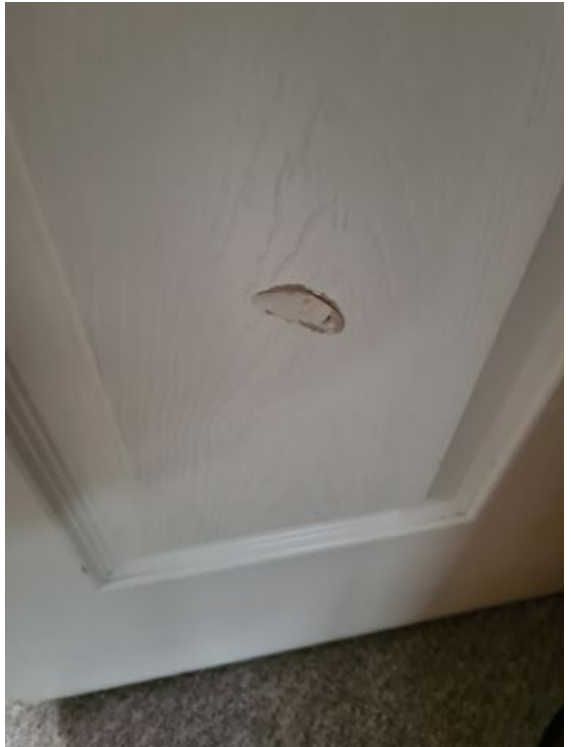
Image 31: INTERIM INSPECTION IMAGES
