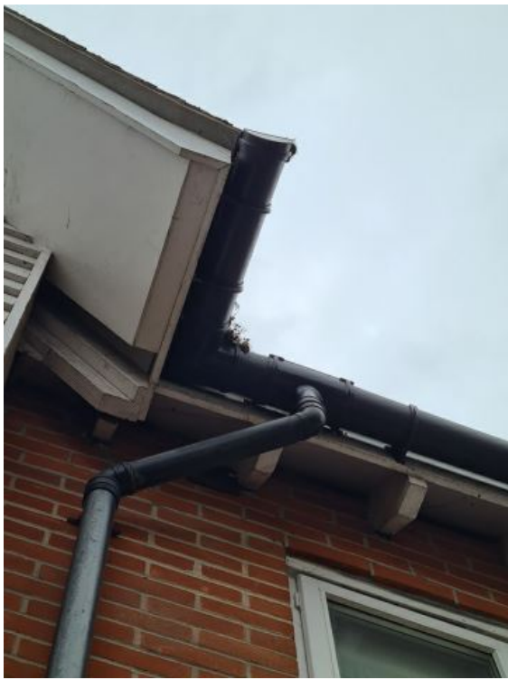
Image 80: INTERIM INSPECTION IMAGES
