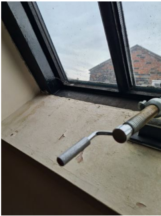
Image 64: INTERIM INSPECTION IMAGES
