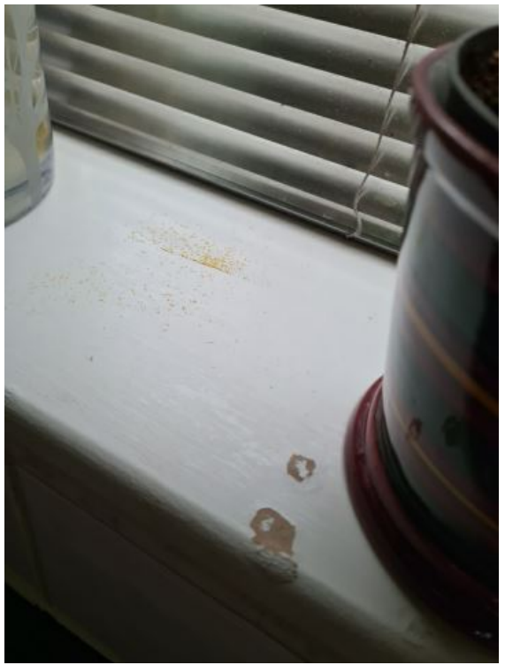
Image 29: INTERIM INSPECTION IMAGES
