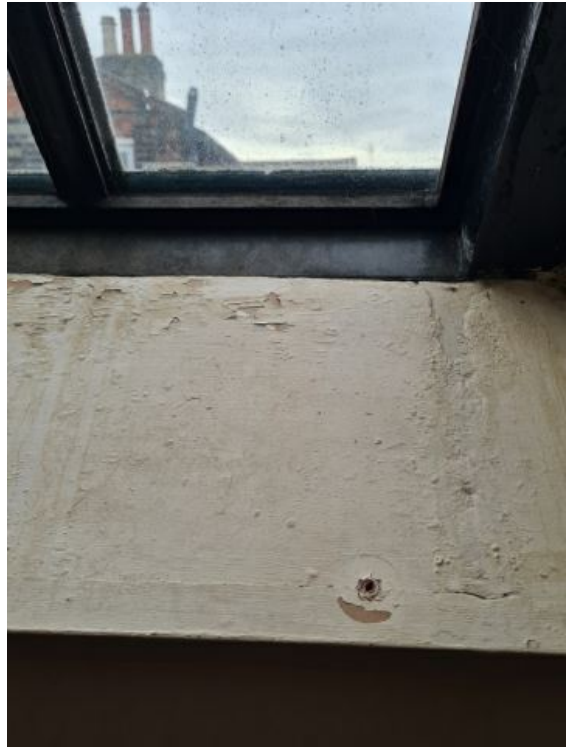
Image 63: INTERIM INSPECTION IMAGES
