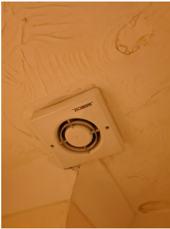
Image 12: INTERIM INSPECTION IMAGES
