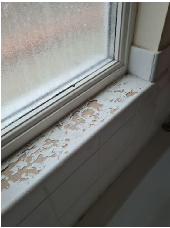
Image 44: INTERIM INSPECTION IMAGES
