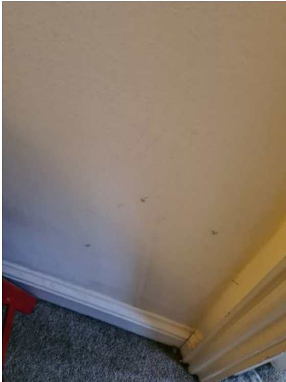
Image 6: INTERIM INSPECTION IMAGES
