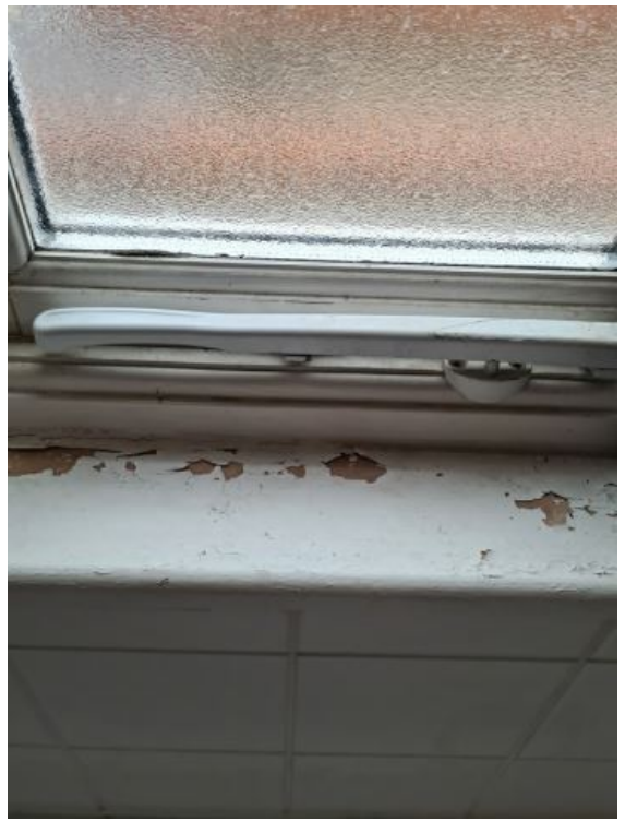
Image 45: INTERIM INSPECTION IMAGES
