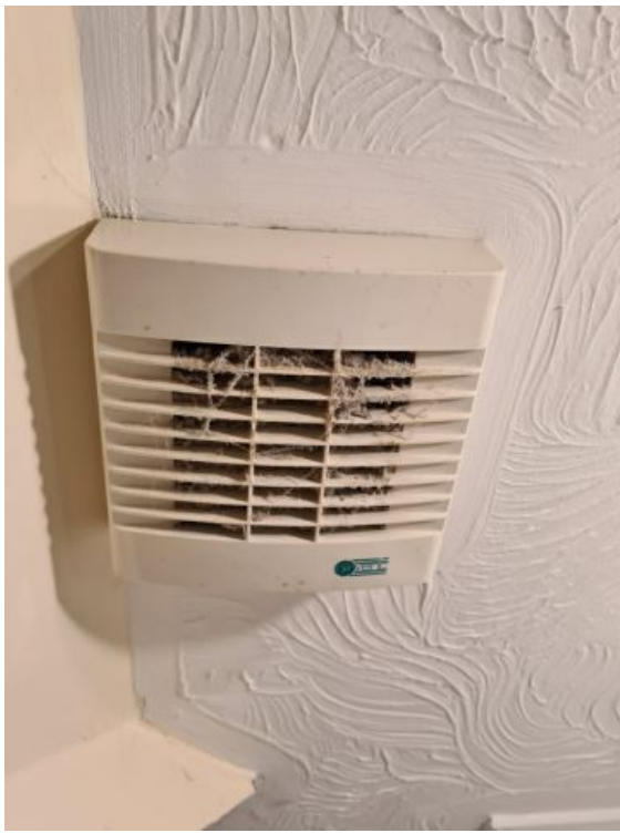
Image 72: INTERIM INSPECTION IMAGES
