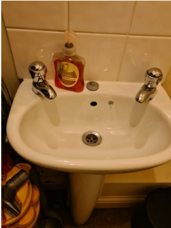
Image 14: INTERIM INSPECTION IMAGES
