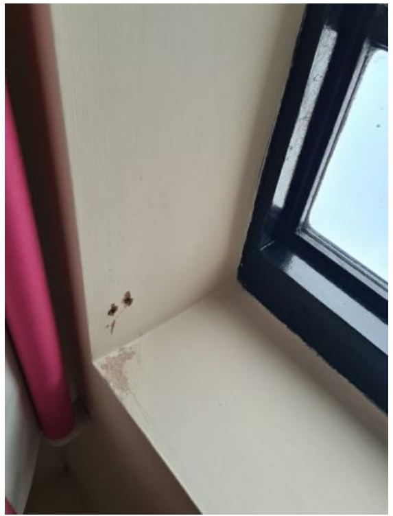
Image 65: INTERIM INSPECTION IMAGES
