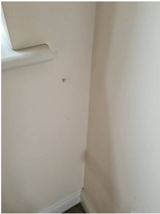
Image 36: INTERIM INSPECTION IMAGES
