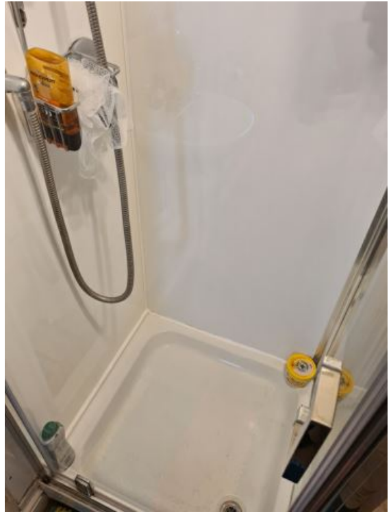
Image 71: INTERIM INSPECTION IMAGES
