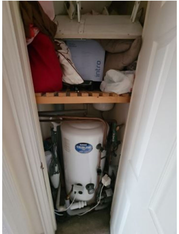
Image 39: INTERIM INSPECTION IMAGES
