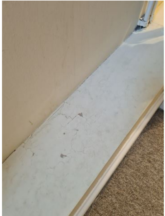
Image 75: INTERIM INSPECTION IMAGES
