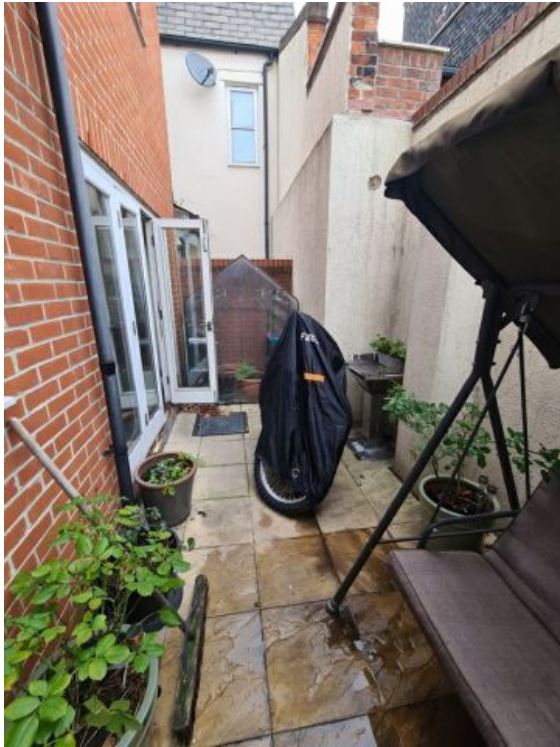
Image 78: INTERIM INSPECTION IMAGES
