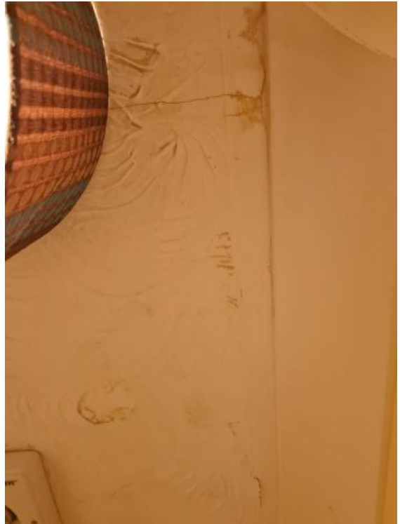
Image 11: INTERIM INSPECTION IMAGES
