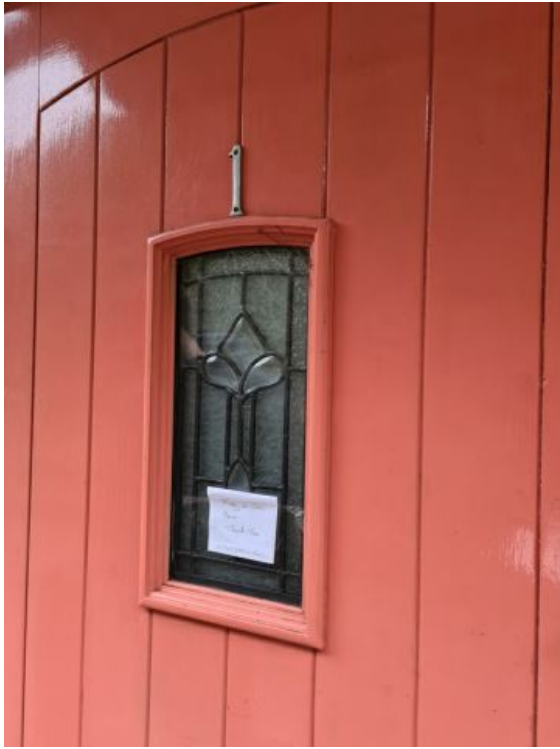
Image 0: INTERIM INSPECTION IMAGES
