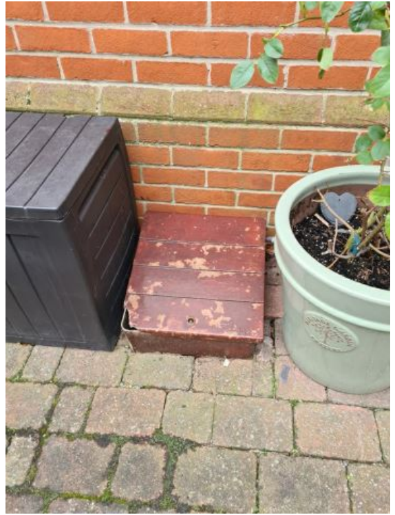
Image 1: INTERIM INSPECTION IMAGES
