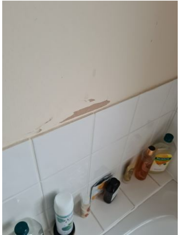
Image 43: INTERIM INSPECTION IMAGES
