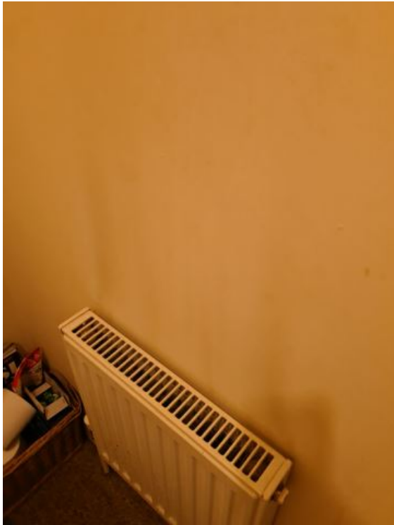
Image 10: INTERIM INSPECTION IMAGES
