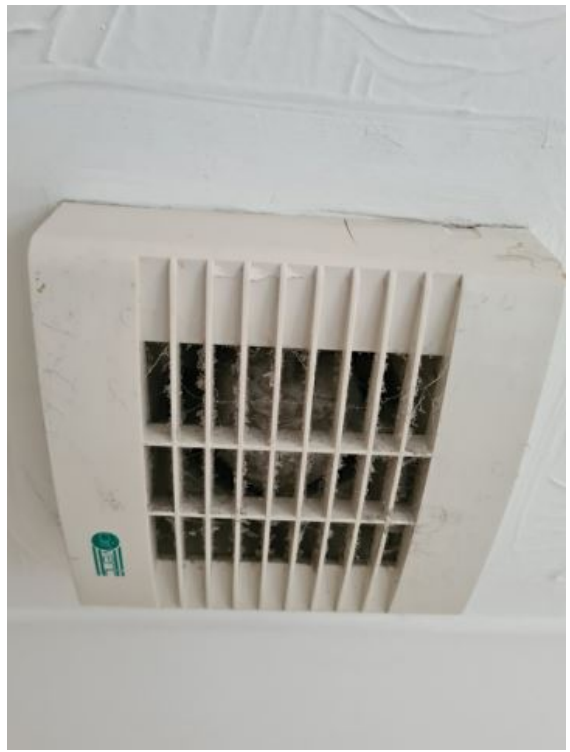
Image 49: INTERIM INSPECTION IMAGES
