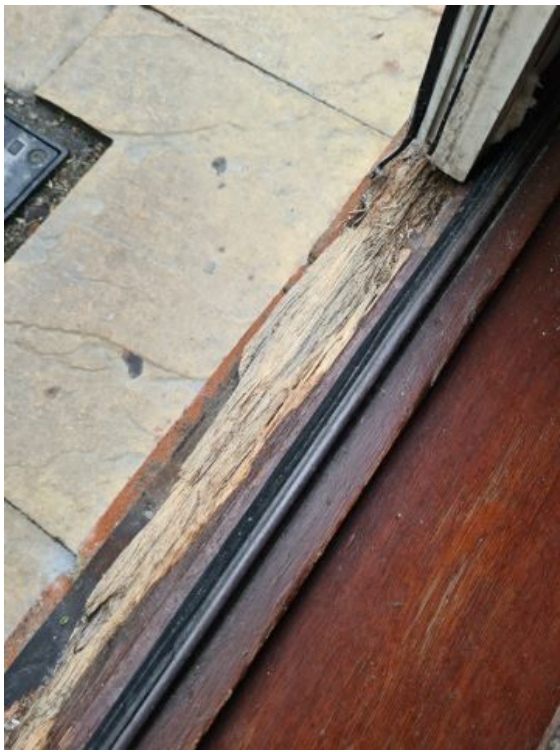
Image 76: INTERIM INSPECTION IMAGES
