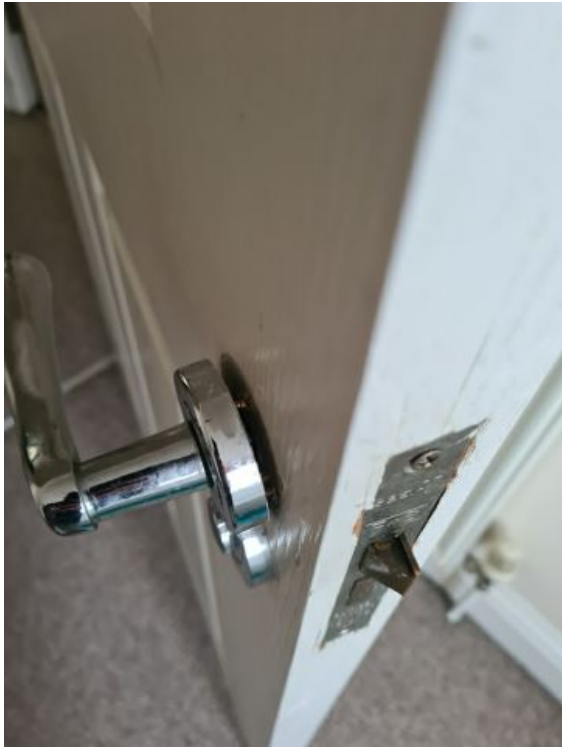
Image 50: INTERIM INSPECTION IMAGES
