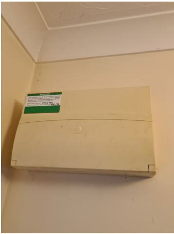
Image 8: INTERIM INSPECTION IMAGES
