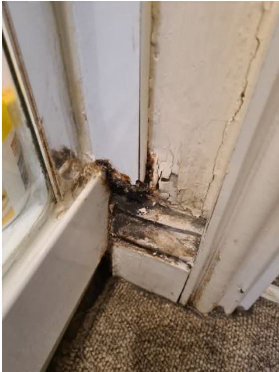
Image 70: INTERIM INSPECTION IMAGES
