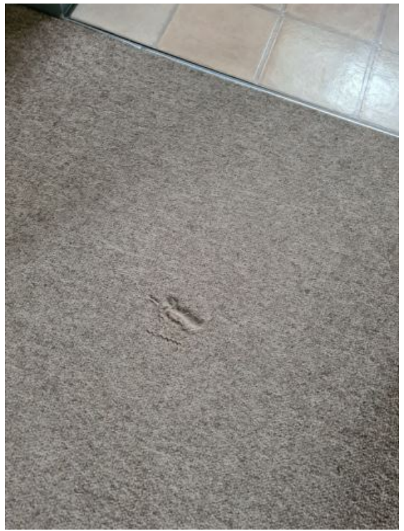
Image 21: INTERIM INSPECTION IMAGES
