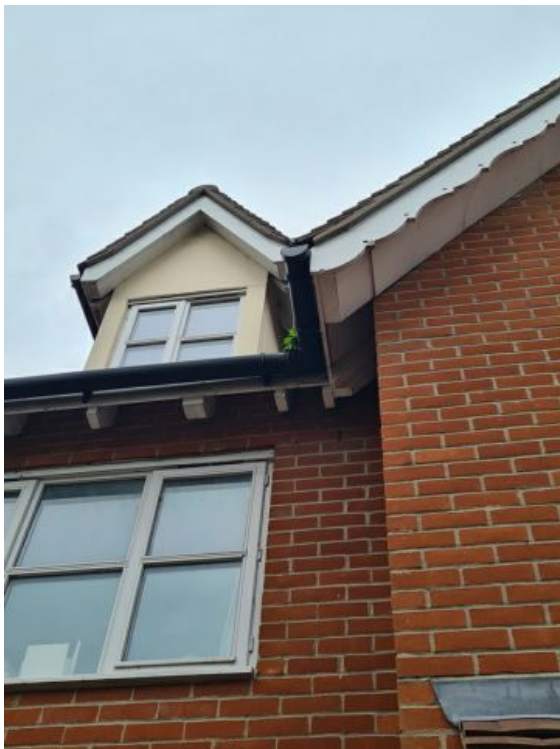
Image 2: INTERIM INSPECTION IMAGES
