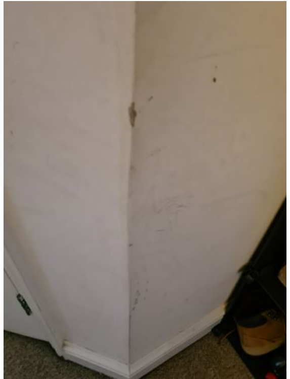
Image 7: INTERIM INSPECTION IMAGES
