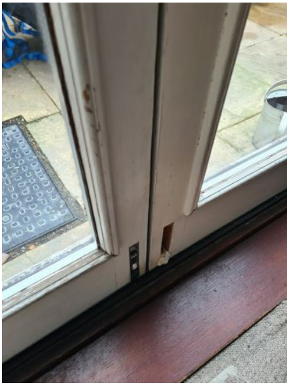
Image 20: INTERIM INSPECTION IMAGES
