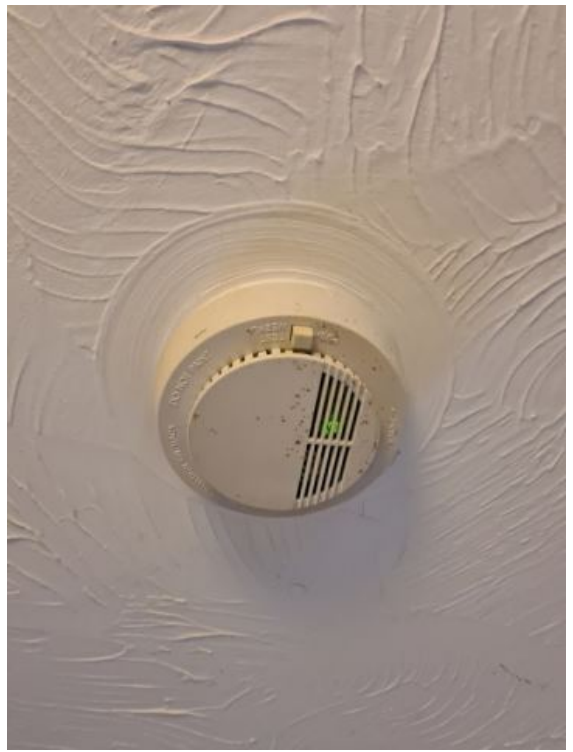
Image 5: INTERIM INSPECTION IMAGES
