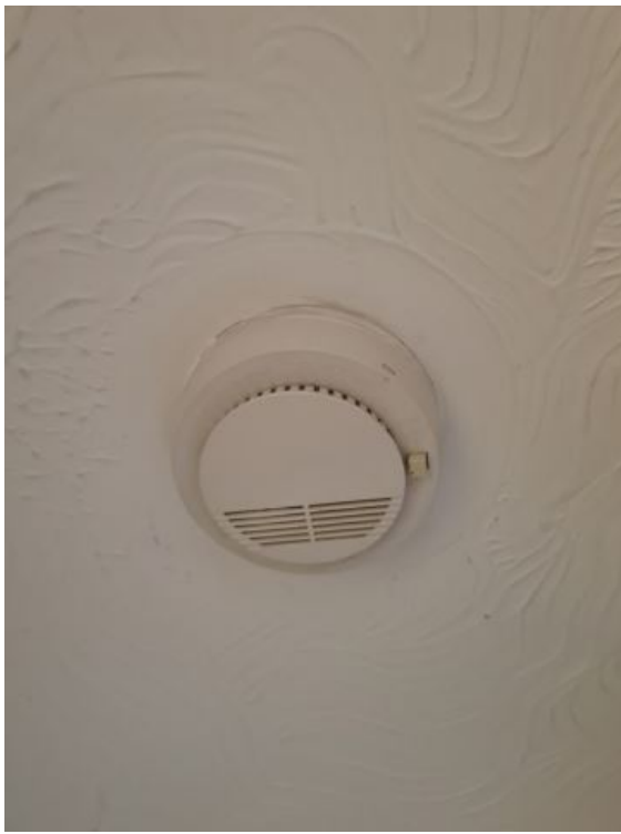
Image 60: INTERIM INSPECTION IMAGES
