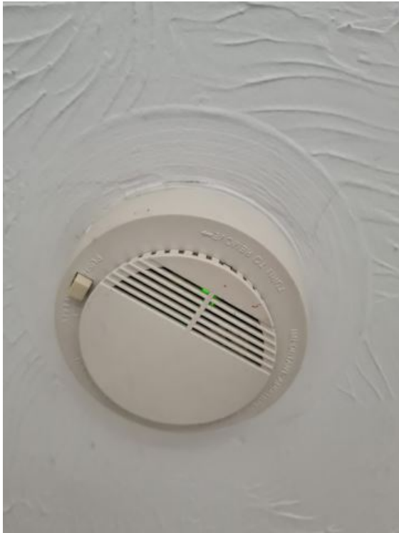
Image 38: INTERIM INSPECTION IMAGES
