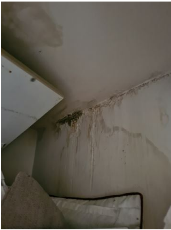
Image 40: INTERIM INSPECTION IMAGES
