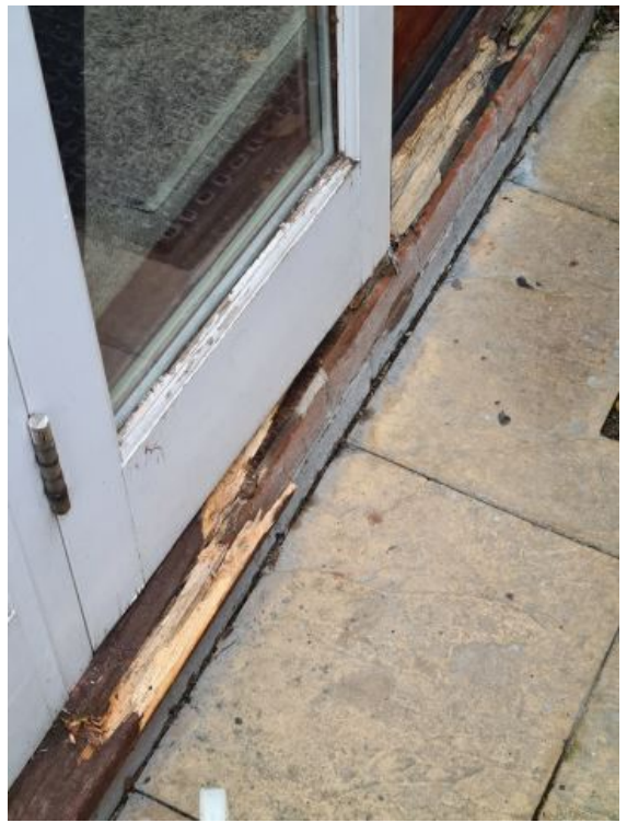
Image 81: INTERIM INSPECTION IMAGES
