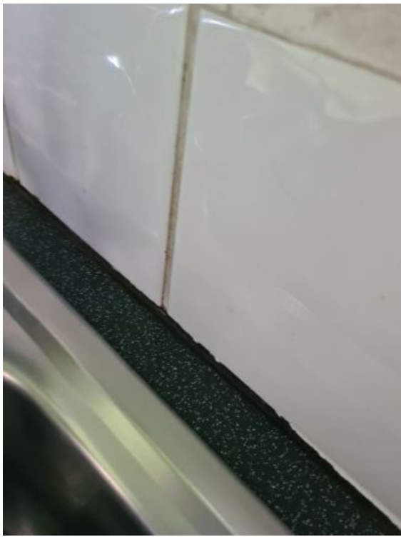
Image 28: INTERIM INSPECTION IMAGES
